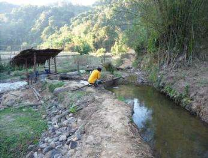
Side channel cut for turbines to be located in
