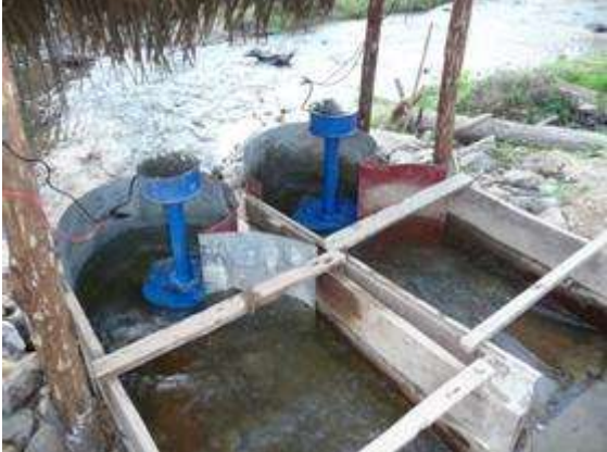
Two new turbines installed in Ansang
